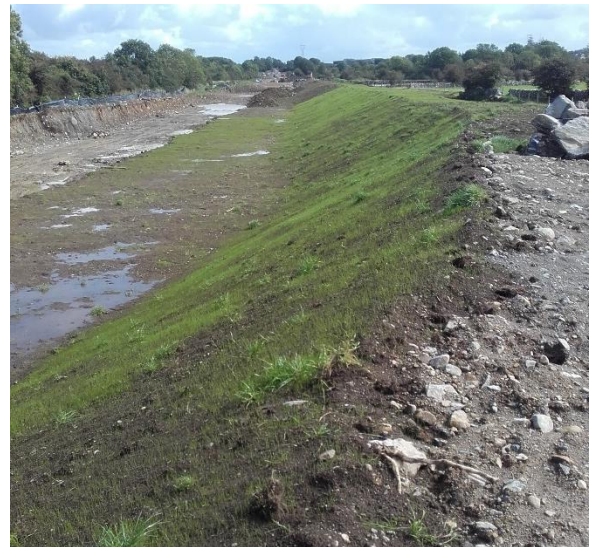
Figure 3a & 3b; Second Stage Channel Formation & Embankment Construction
