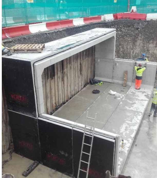
Figure 2; Culvert Installation
